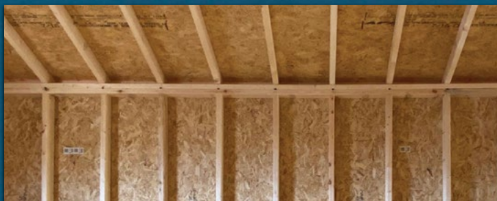
16" ON CENTER TRUSSES (PAINTED ONLY) | F1 16" on center studs are standard
