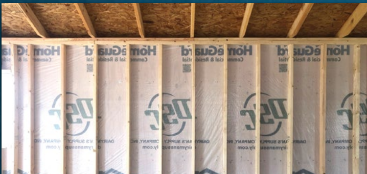
HOUSE WRAP VAPOR BARRIER | P1
